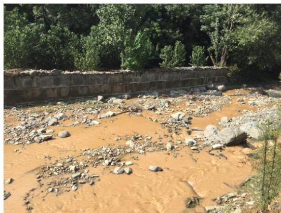
Figure-5.33: A low cost protection bund to control soil erosion and conserve water on stream.
